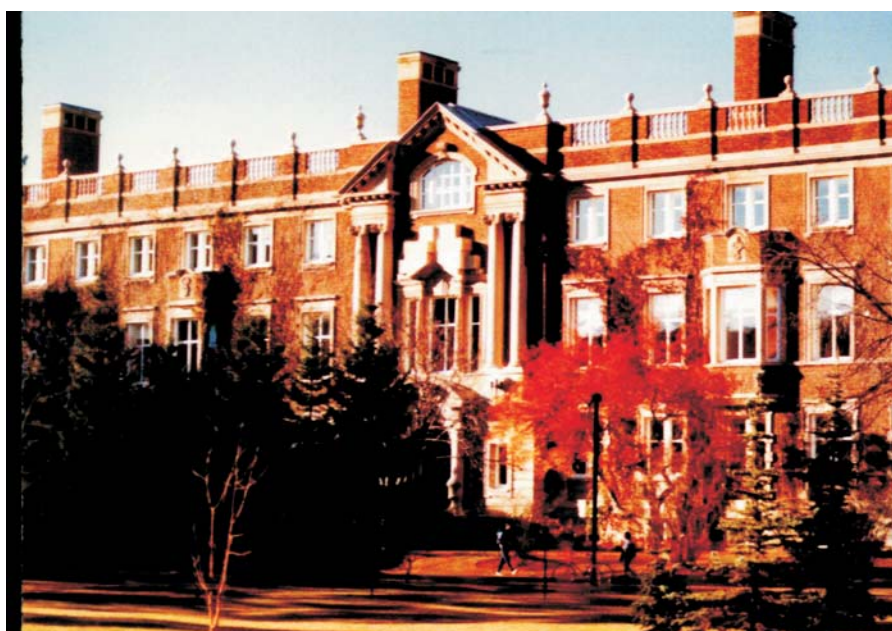
Arts Building at the University of Alberta, location of the Canadian Centre for Austrian and Central European
